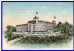
Water Gap House.jpg
